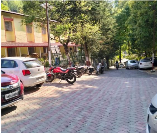
Paving stone installed in campus
