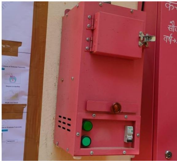
Incinerators installed for BMW management
